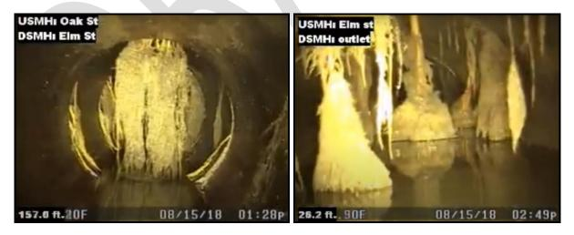
The tree roots have easy access through the joints between the tiles. Root intrusion tends to accelerate more rapidly in dry years when tree roots are following the water in search of moisture. The video inspection was completed five years ago, and especially due to the last few dry years tree root intrusion is expected to be more extensive today.
